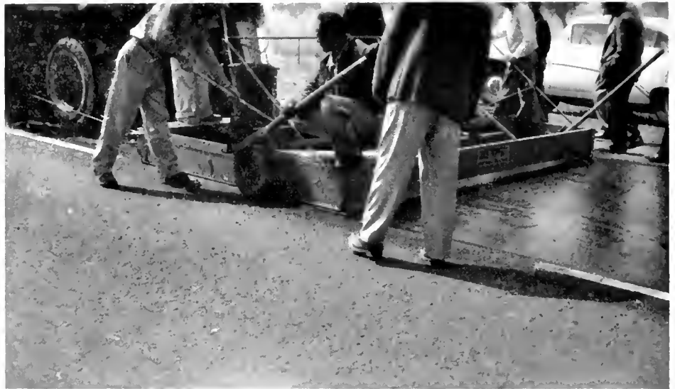
Spreading slurry
